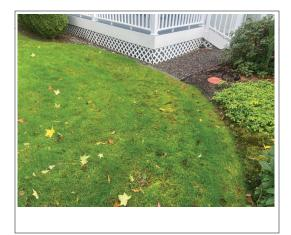
Negative slope observed in some areas around the building. There should be adequate slopes of the land and ground around a property. The slopes of the ground should be directed toward appropriate and approved drainage devices that are capable of carrying concentrated runoff. Current industry standards
