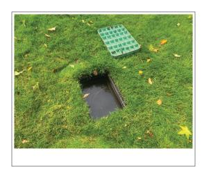
The water meter junction box was approximately 1/2 filled at the time of inspection
